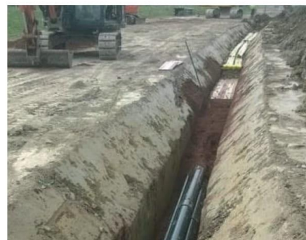
Laying the ducts
