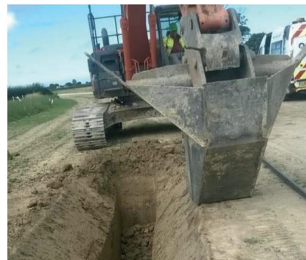
Excavation of the cable trench
